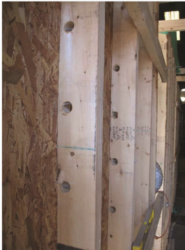
Figure 2 - Observation holes at anchoring screws in wood studs.
