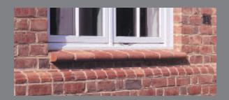
angular or curvilinear, add distinctive detailing to wall caps, windows, and door openings. Tread shapes are manufactured to properly finish brick steps and other paving applications.
