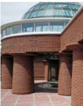
Dimensions for Glen-Gery's standardized radial brick are computed so that the arc length appears equal to the length of the accompanying stretcher units. They are also designed so that a whole number of brick fall within a 90° segment, eliminating the need to cut brick to achieve tangency at 90°, 180° or 270°.
