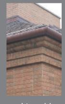
these shapes can be used to add dimension to flat walls, rotated to form door and window jambs, or inverted to form cornice brickwork. Continuity of design can also be transferred into the landscape by using the water tables as caps for walls or edging accents for walkways.
