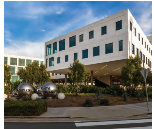
The Brickyard, Aspen White Thin Brick - Precast installation
